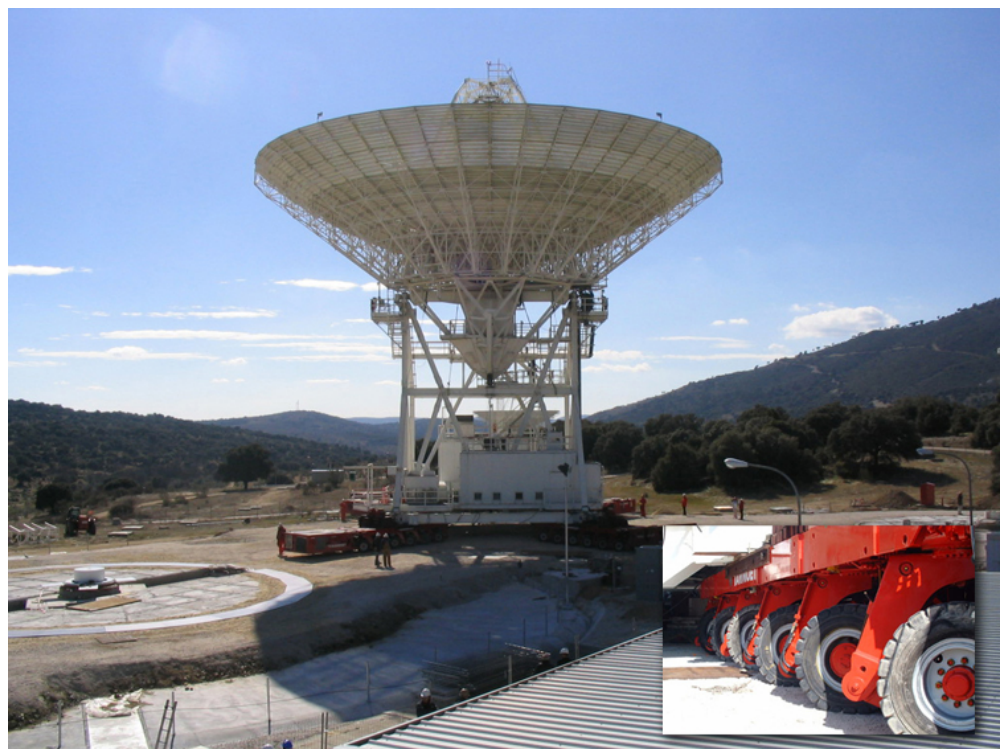
Giant Deep Space Network antenna in Madrid is moved using four 12-axle, 24-wheel crawlers.
