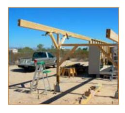
The roof is supported by 4-inch rollers, 5 on each wall/rail. The 2x4 rafters are on 12-inch centers for rigidity. The roof is standard construction of chip board, felt and composition shingles. It is heavy, but still manageable
